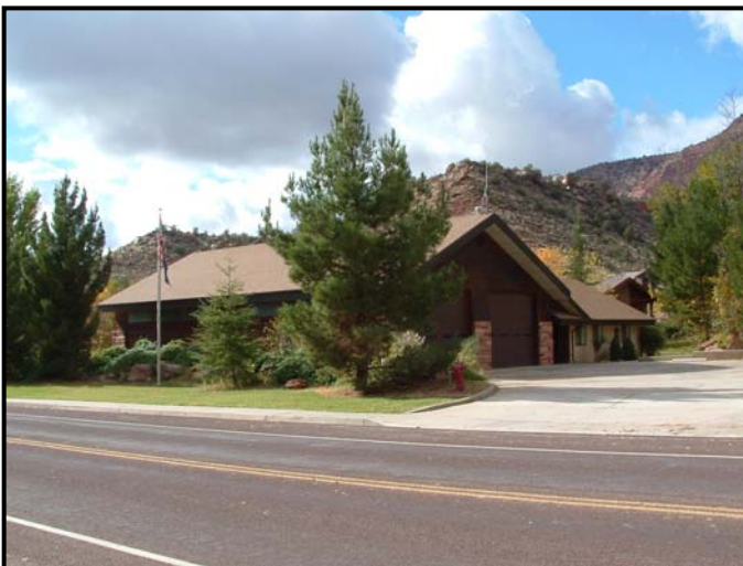
Picture 1 – Fire Station in Springdale
