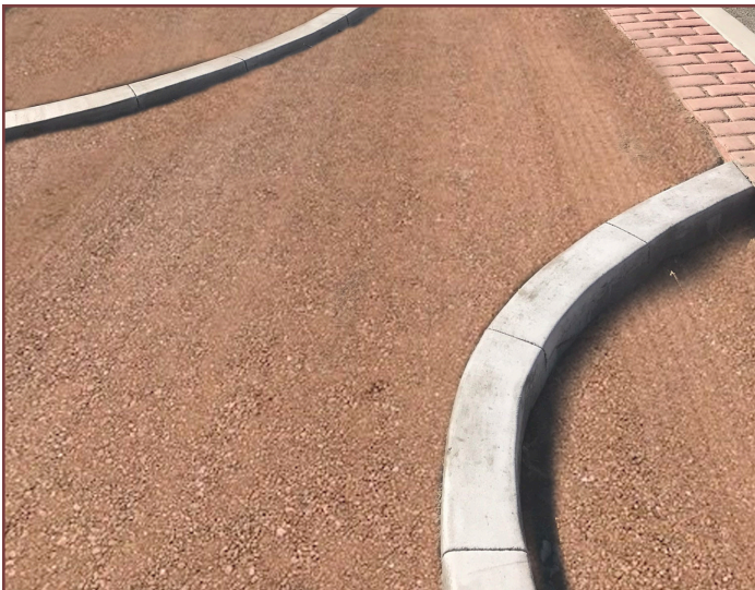
Decorative Ribbon Curb
