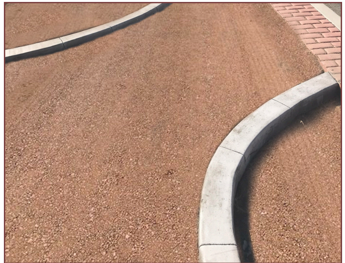
Decorative 6" Ribbon Curb
