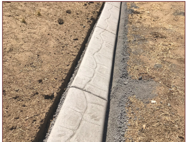
Decorative Ribbon Curb
