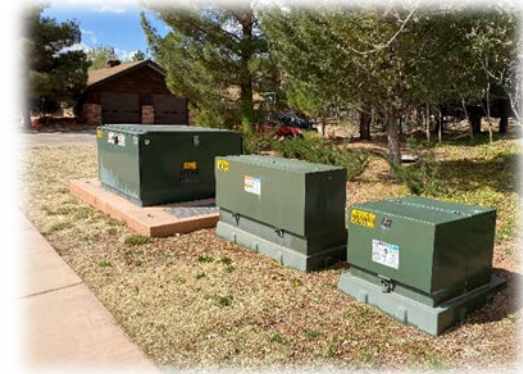
North of the Fire Station
