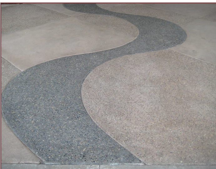
Sandblasted & Stained Pattern in Pavement
