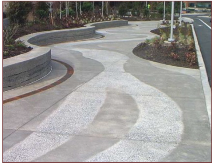
Sandblasted Pattern in Pavement
