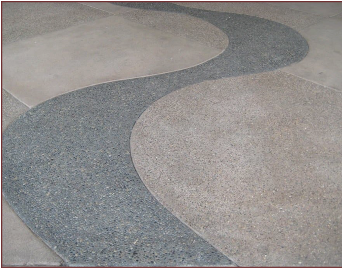
Sandblasted & Stained Pattern in Pavement
