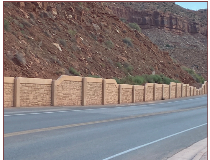
Existing Retaining Walls
