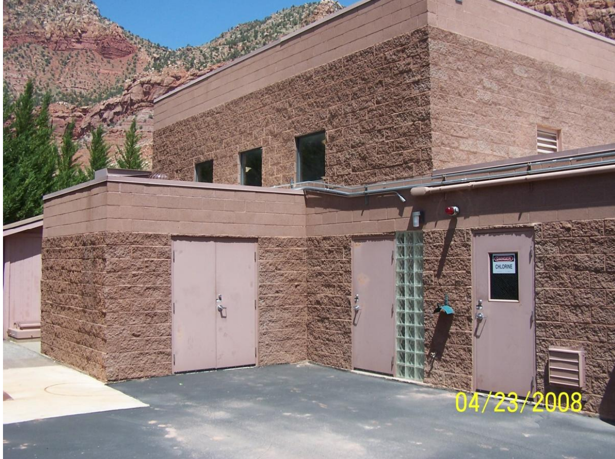
Figure V-1: Existing Springdale Water Treatment Facility
