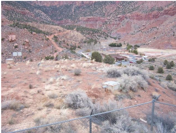
Figure IV-2: North Concrete Tank
