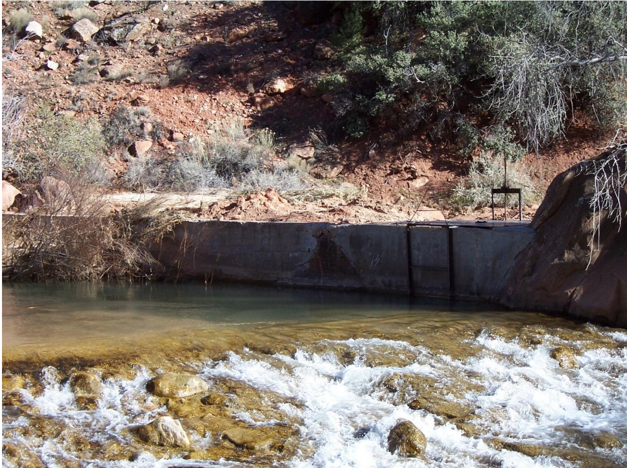
Figure III-1: Existing Virgin River Intake Structure
