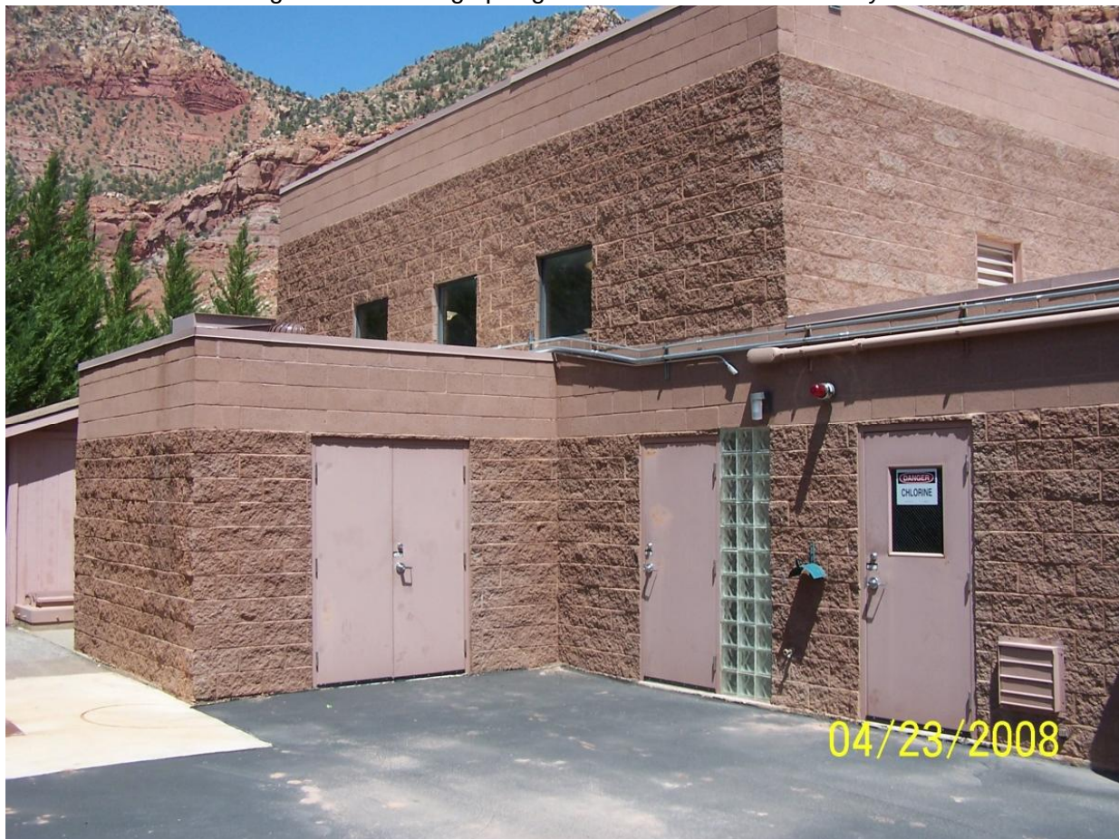
Figure I-1: Existing Springdale Water Treatment Facility
