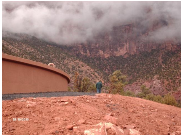
Figure IV-3: 1MG Concrete Tank
